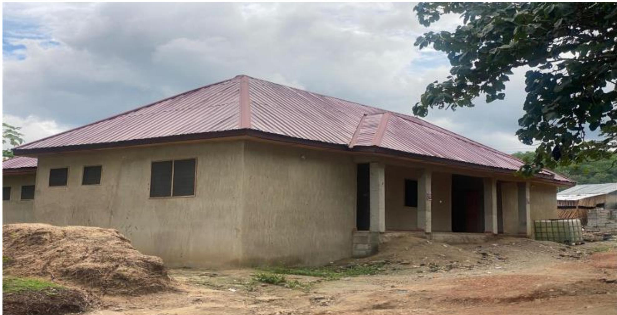
CONSTRUCTED IMPROVED 1NO. 16-SEATER W/C TOILET FACILITY WITH 4NO. BATHROOMS, 6NO. URINALS WITH 4000LT SEPTIC POLYTANK WITH CONCRETE STORAGE TANK AND 1NO. 2000LT OVERHEAD POLYTANK CONNECTED TO ELECTRICITY AT ABONO-TILING LEVEL
